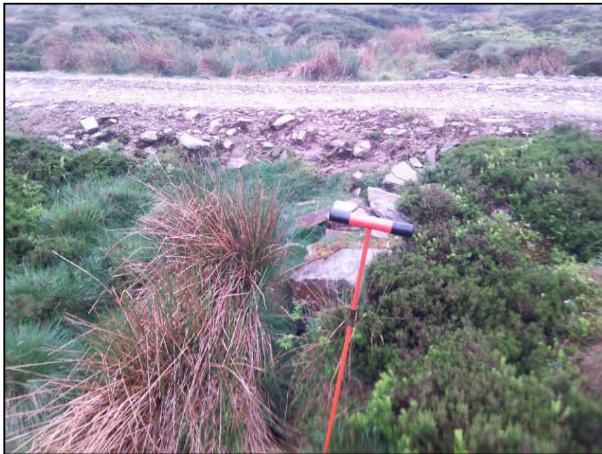
Photo 20 T20: Artificial trackside drainage Easting, Northing (278329, 821554)
